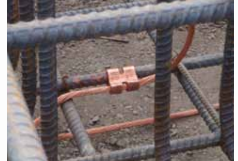
Grounding wire to rebar
