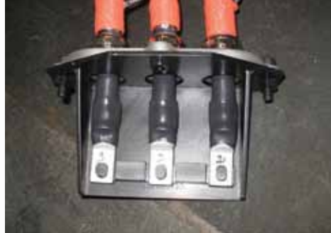
Grounding wire to steel
