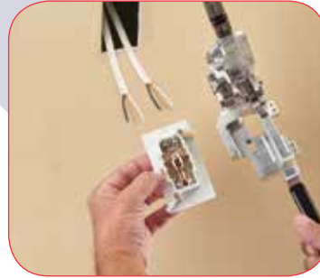
1 Prepare wire and place device into the tool cradle.
