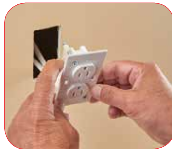
7 Push device into the wall and tighten pawls.
