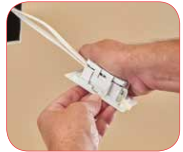
6 Snap-on the cover into the device.
