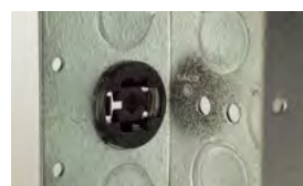
Step 2: Done - Ready for cable.
