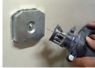
3. Devices and wiring are now protected from router bit, drywall mud, and paint
