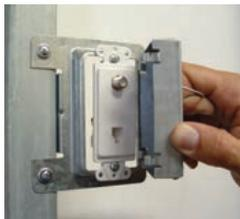
2. Snap protection plate on to data ring. Ring is ready for drywall.
