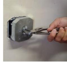
4. Remove cover using tab with lineman plier or Channel-locks™.
