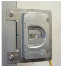
2. Snap protection plate on to data ring. Ring is ready for drywall.
