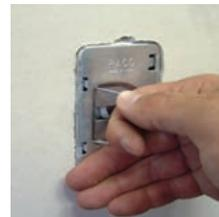
4. Using finger pull, remove protection plate and finish termination.
