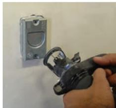
3. Device and wiring are now protected from router bit tool, drywall mud, and paint.
