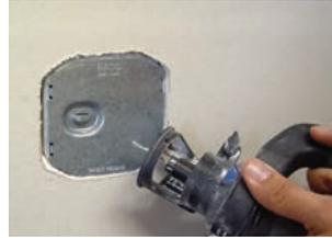
3. Wiring is now protected from router bit, drywall mud and paint.
