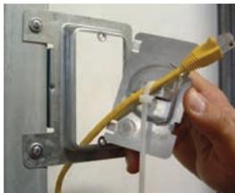
1. Install low voltage ring. Secure cable to back of protection plate using cable tie.
