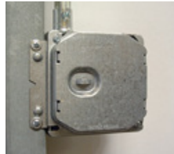
2. Snap protection plate on mud ring. Box is now ready for dry wall.
