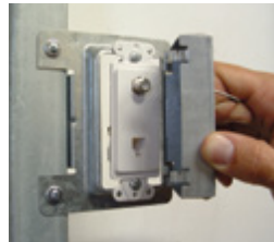
2. Snap protection plate on to data ring.
