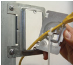
1. Data ring attached to stud with string or cable secured to protection cover.
