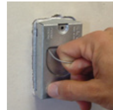
4. Using finger pull, remove protection plate and finish termination.
