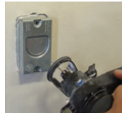
3. Device and wiring are now protected from router bit, dry wall mud, and paint.
