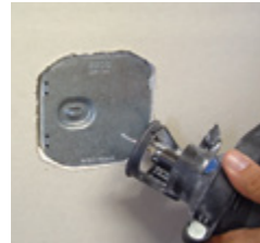
3. Wiring is now protected from router bit, dry wall mud, and paint.
