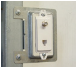
1. Data ring with device installed.
