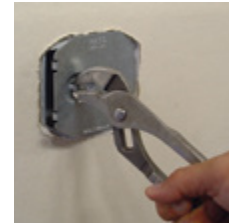
4. Remove cover using tab with lineman plier or Channel-locks™.
