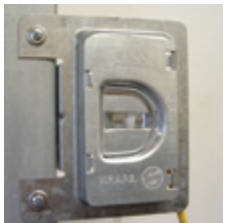
2. Snap protection plate on to data ring.
