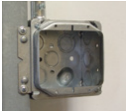
1. Box, mud ring mounted to stud.
