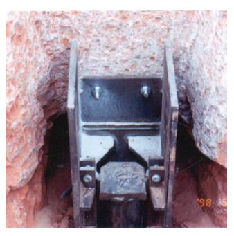
Close-up view of the installed pier. The Atlas Resistance® Pre-Drilled Pier System is constructed of 1/2" and 3/4" steel for heavy-duty applications. The assembly weighs nearly 300 pounds and has an ultimate capacity of 76,000 pounds!
