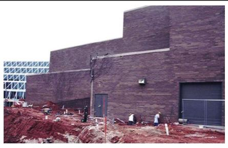
Above is a view of the job site where workers are installing supplemental support. Atlas Resistance® Pre-Drilled Piers provided support to the existing structure during excavation.
