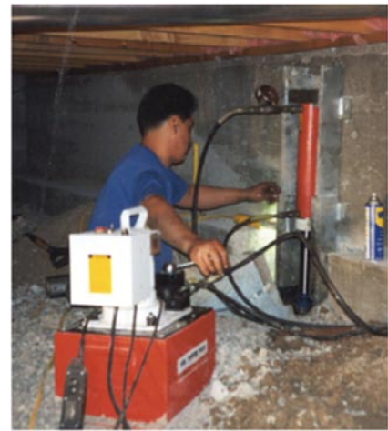
Notice how the footing was notched to allow the Atlas Resistance® Pier to be installed as close to the stem wall as possible.
