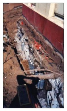
support the design load of 40,000 pounds per anchor with a safety factor of two.
