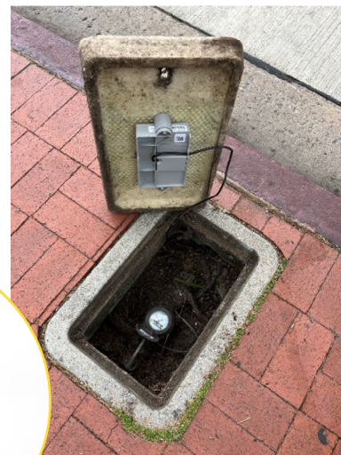
Aclara MTU positioned on the underside of an Armorcast lid
