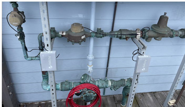
Completed installation of Aclara MTUs
