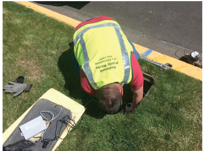
Aclara MTU being installed in Redmond.
