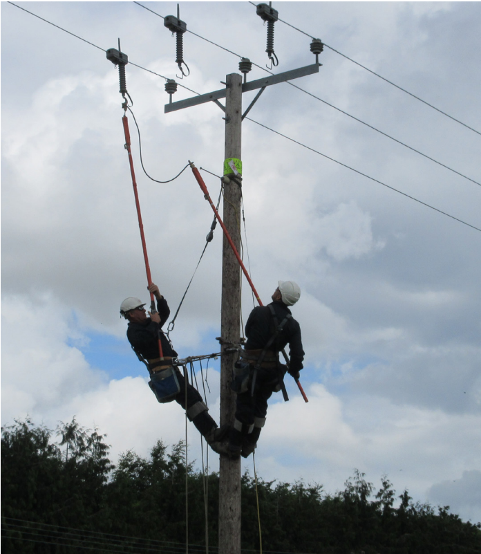
Power sensors are installed on overhead lines with hot sticks and require no calibration or additional, pole-mounted equipment.
