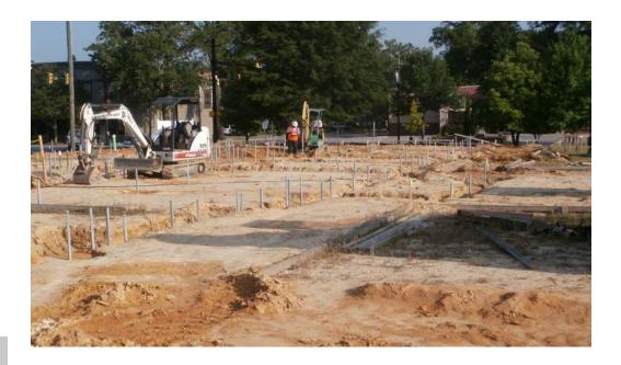
66 While the contractor could dig down about two feet, no spoils could be generated, which is why yje design called for helical piles.
