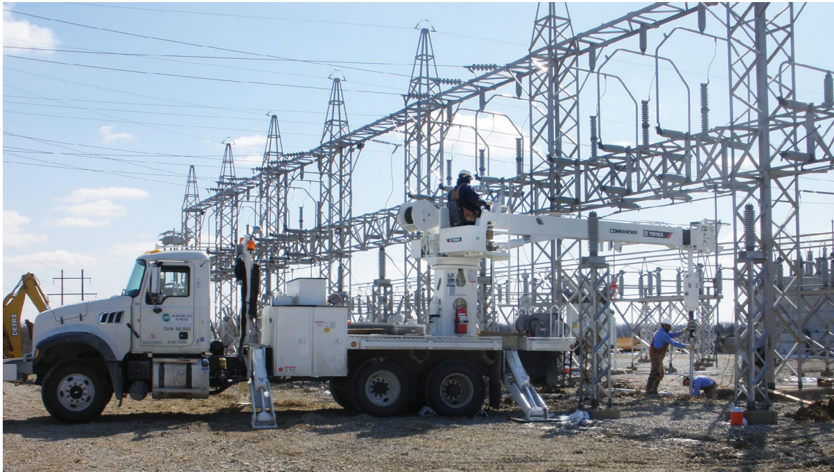
Workers drive in helical piles to augment a 69-kV tower foundation at Henry substation. Helical piles were the only way to go on this project. The work had to be completed in tight quarters, on a short deadline and while the substation was still energized.
