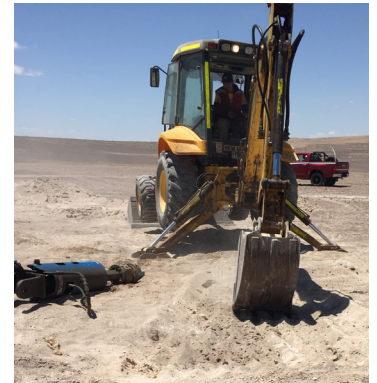
The Caliche soil is very dense so digging is difficult, even with a backhoe
