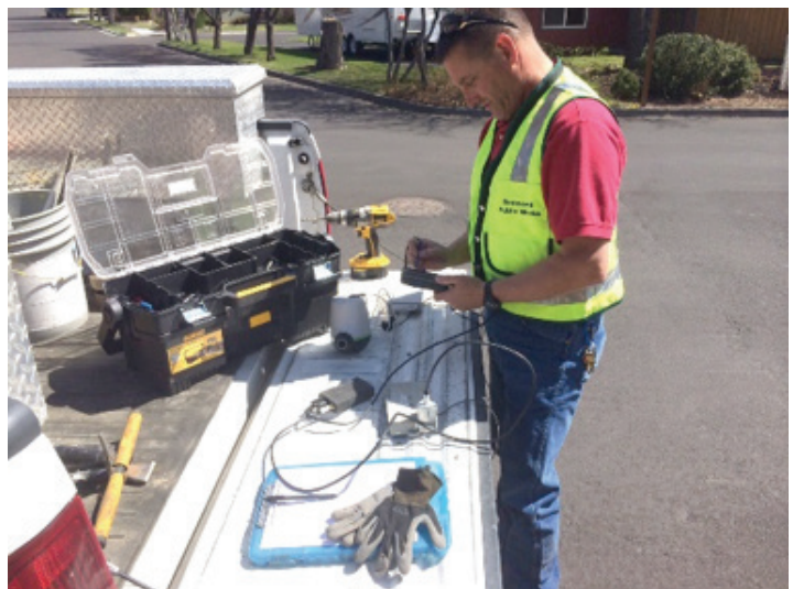
Preparing MTUs for installation.
