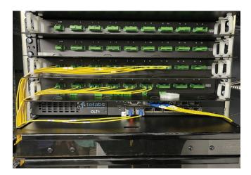
Hubbell FCR-X series fiber enclosure manages fiber to the Tellabs FlexSym OLT while Hubbell 2:16 rackmounted 1U splitters with custom-length assemblies distribute connectivity from the OLT to tech lockers that serve passenger cabins.
