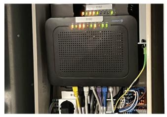
ONTs housed in tech lockers provide technology for passenger cabins via Hubbell's NEXTSPEED Ascent Category 6A shielded cabling, color-coded for straightforward application identification (Wi-Fi, phones, TVs, lighting control, etc.).
