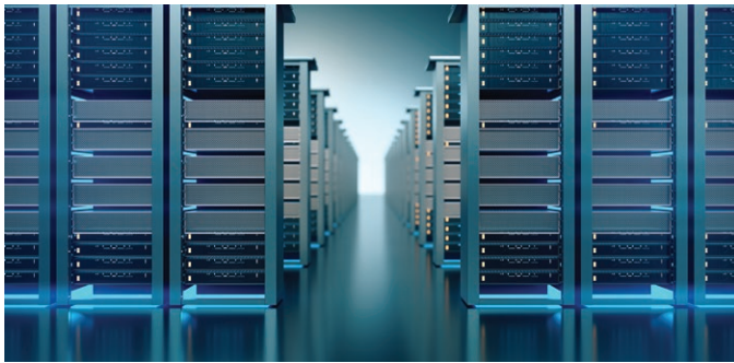
Figure 5: AHFs at the server room in the second floor
