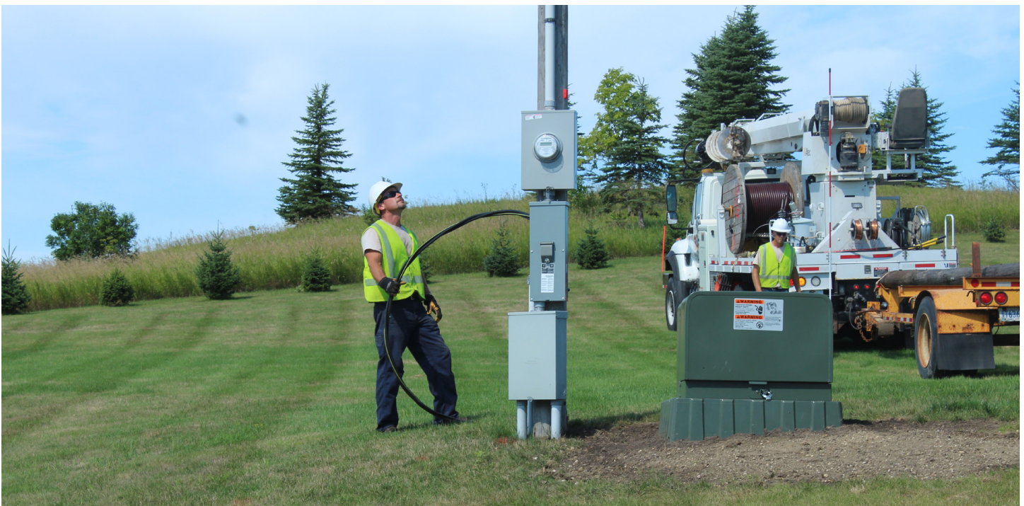
Fig. 1 - The rural nature of the Runestone Electric Association service area, with low meter density per square mile, made TWACS the best choice for the utility because it operates on existing power line infrastructure.
