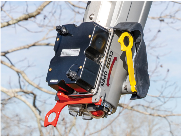
Fig. 3 – Manual open/close operation via yellow handle and visual open/closed status via mechanically-linked semaphore
