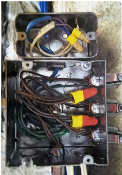
A: Class 2 wires in separate enclosure
