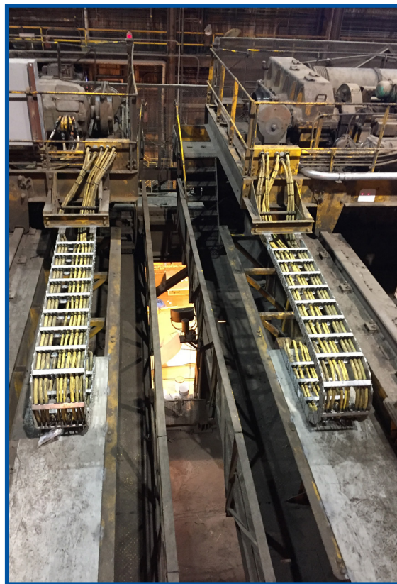
Steel Carrier in Mill Application
