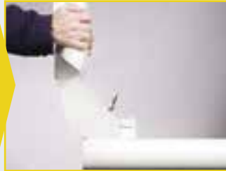
SLIDE LUMINAIRE ONTO SPEED MOUNT AND SECURE
