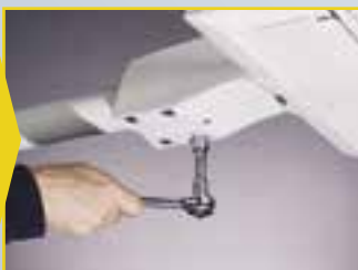
ADJUST BOLTS TO SECURE LUMINAIRE
