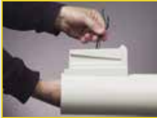
INSTALL SPEED MOUNT, FISH WIRE THROUGH POLE AND SPEED MOUNT
