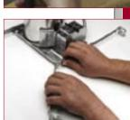
Pro-Nail bar hangers can be quickly and easily reoriented 90° on the plaster frame to avoid obstructions or to reorient the junction box.
