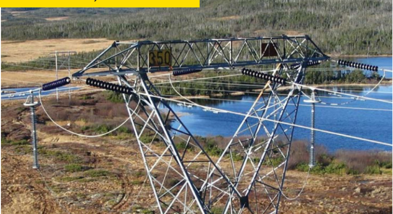
230kV - Manitoba, Canada
