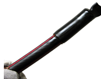
3. HSIC-FR end cap installed on cable.
