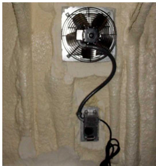
Complete Exhaust Fan (Interior View)
