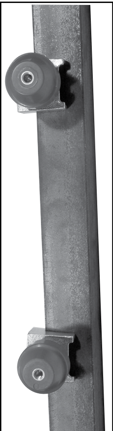
Isolators and mounting hardware remaining after ground bar has been stolen.
