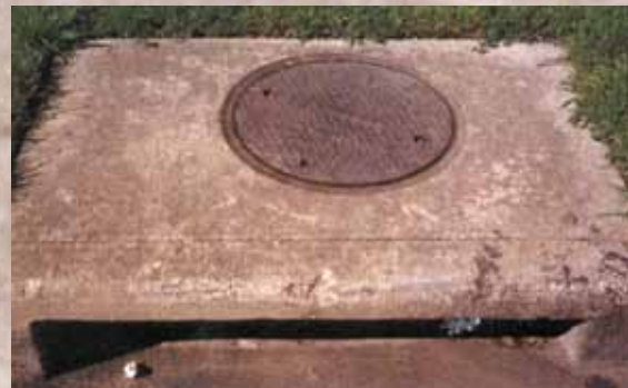
Custom covers can be retrofit to existing frame
