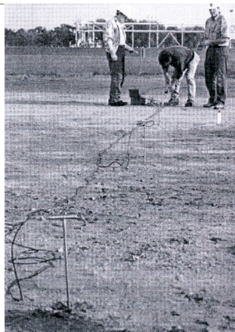
SENSOR PIN INSTALLATION FIGURE A-10
