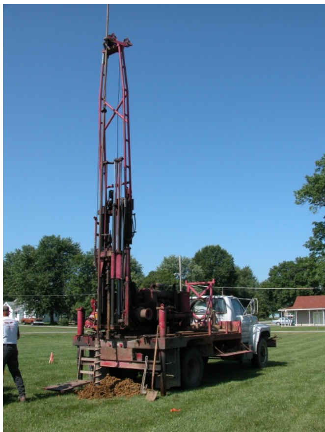
AUGER DRILLING OPERATION FIGURE 2-7
