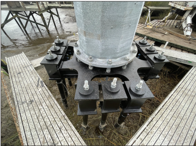
Sacrificial Anode Protection System Figure A-14
