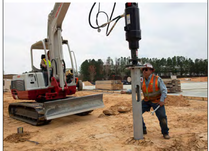
INSTANT FOUNDATIONS ARE INSTALLED USING COMMON CONSTRUCTION EQUIPMENT FIGURE 10-3
