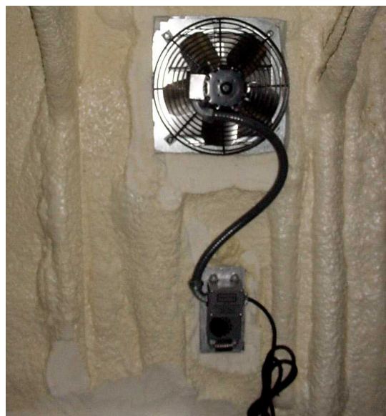
Complete Exhaust Fan (Interior View)
