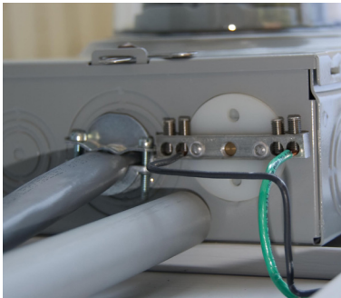
CONFIGURATION 1 - MOUNTED TO ENCLOSURE
