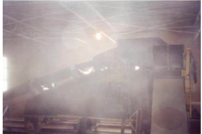
Typical Class II Dust Location
