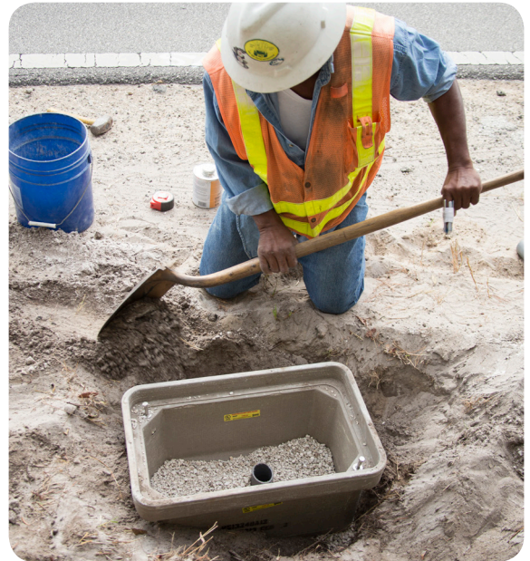
Backfill in 6-inch intervals, manually tamping to ensure backfill gets into channels and ribbing in sidewall of enclosure.
