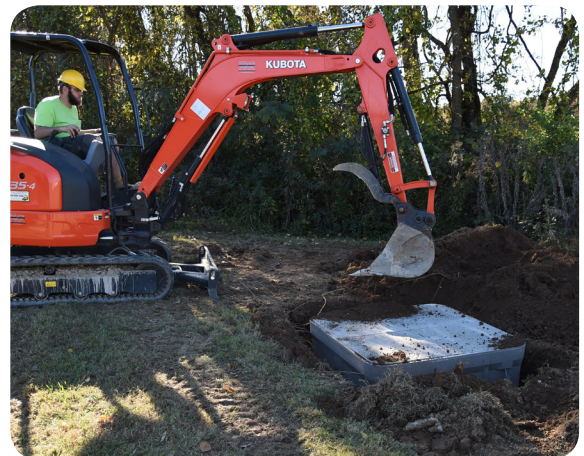
Backfill in 6-inch intervals, manually tamping to ensure backfill gets into channels and ribbing in sidewall of enclosure.
