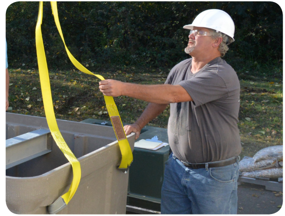
Attach nylon straps or chains to the lifting bolts.
