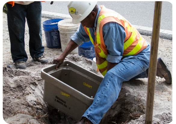
Lift and position enclosure with backhoe.
