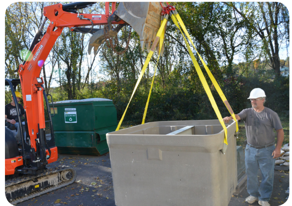
Lift and position enclosure with backhoe.
