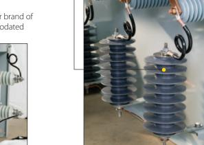
Choose group fusing or individual capacitor fusing, expulsion or current limiting fusing; coordinated with capacitor case rupture curves.
