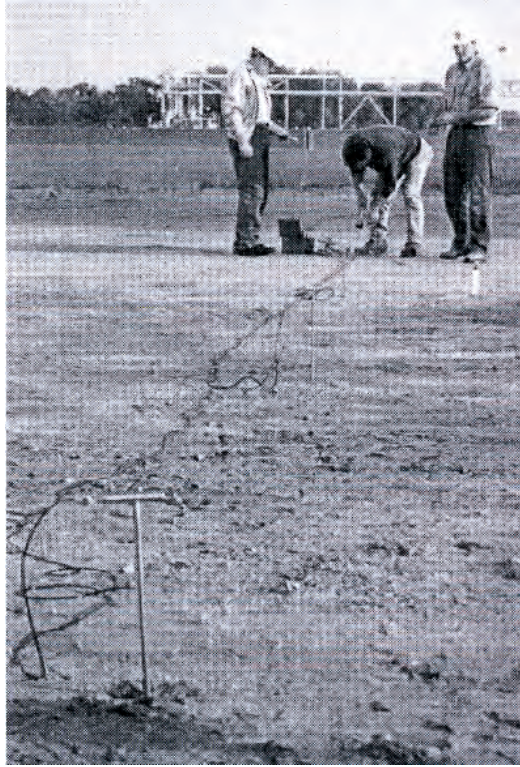
Sensor Pin Installation Figure A-10
