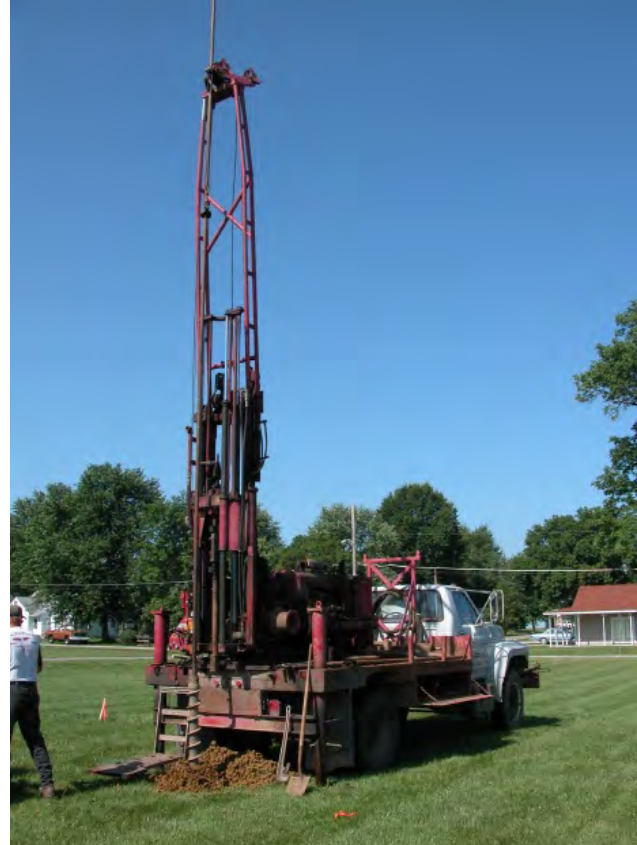
Auger Drilling Operation Figure 2-7
