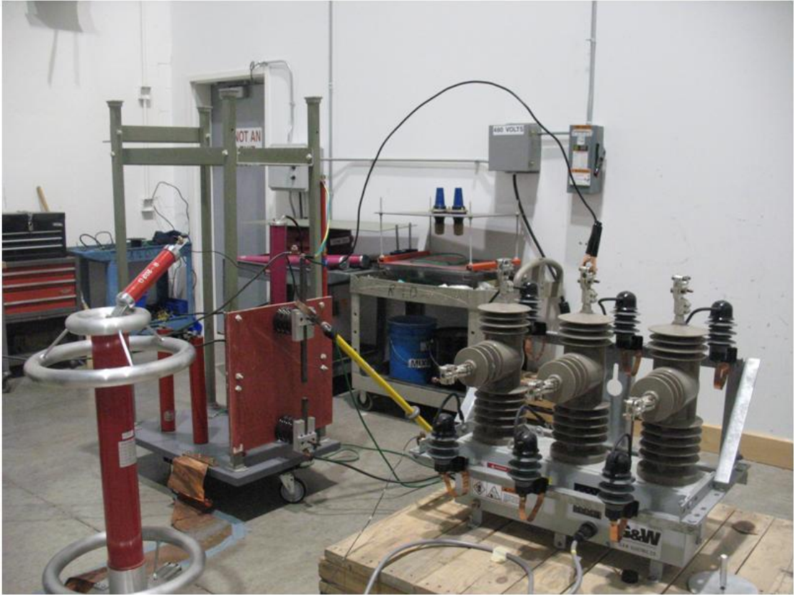
SSAO recloser setup
