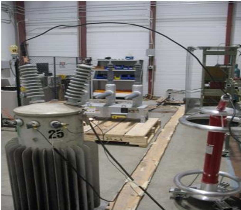
SSAO Transformer Setup
