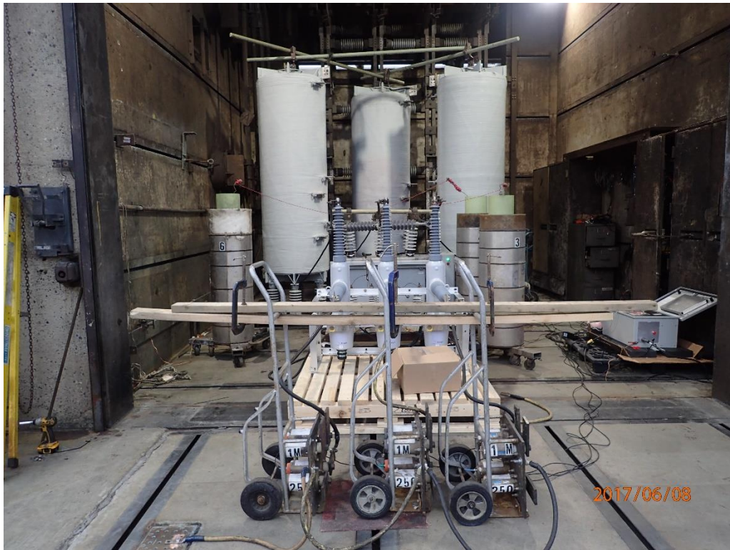
Figure 19: Setup of rated symmetrical interrupting current tests, Duty T100 and T50.
