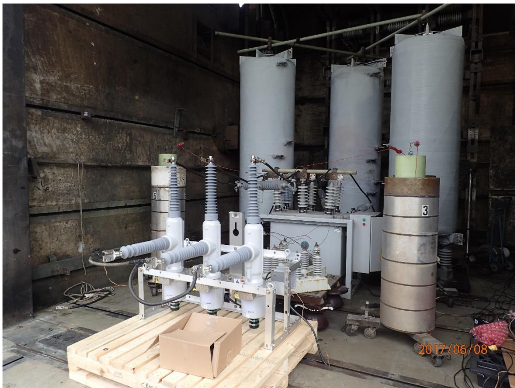
Figure 20: Setup of rated symmetrical interrupting current tests, Duty T20.
