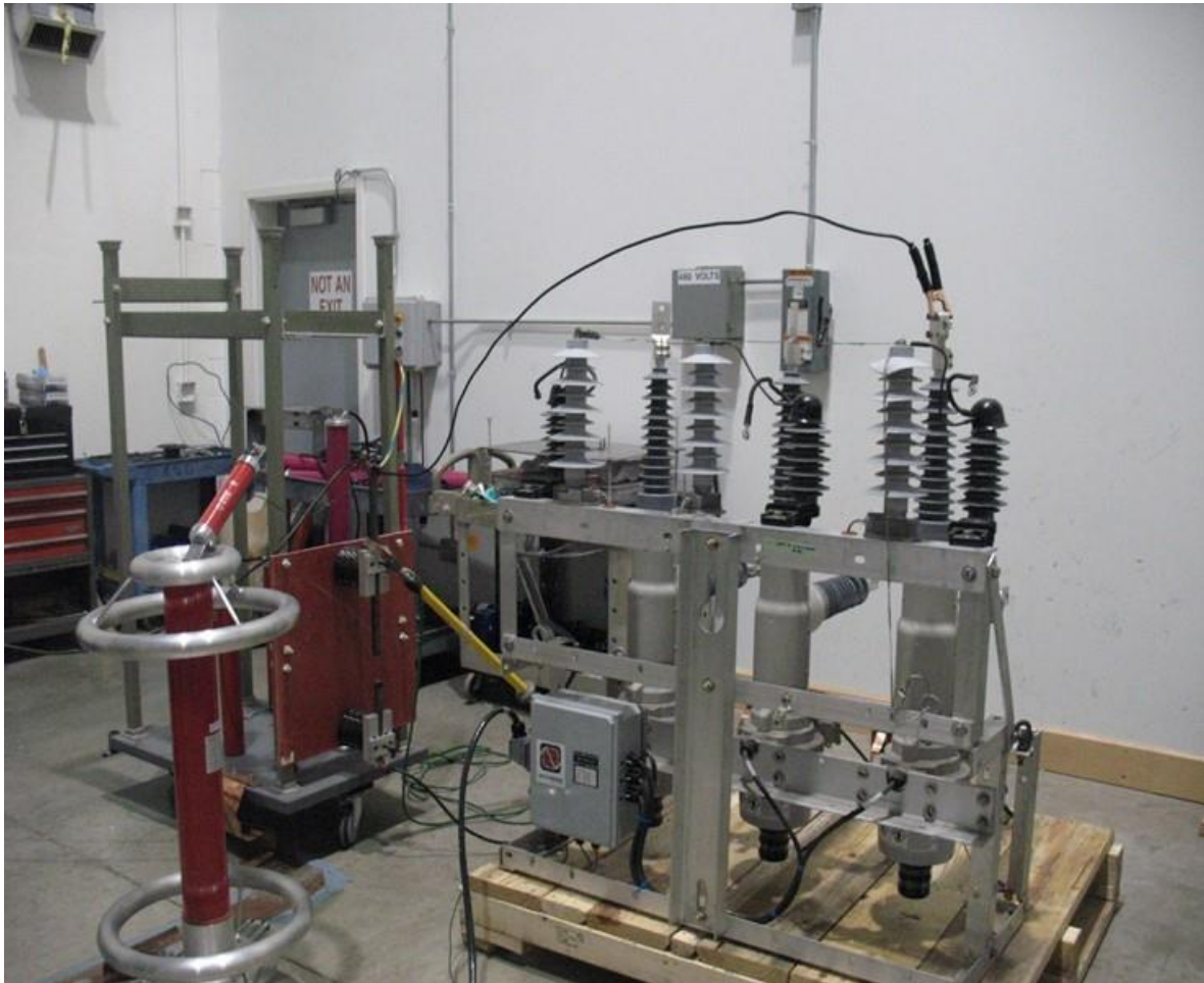
SSAO Recloser test setup
