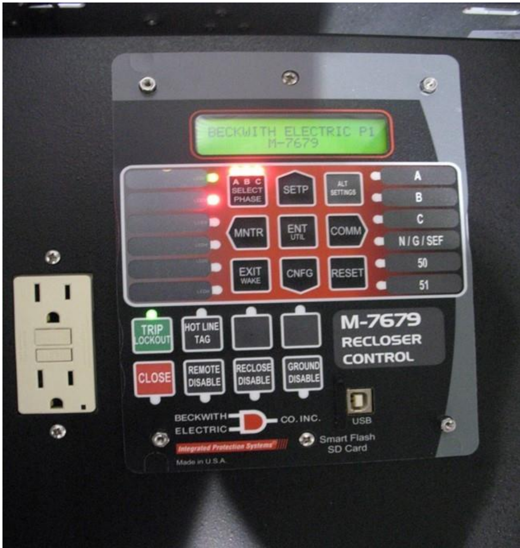
Beckwith control screen display
