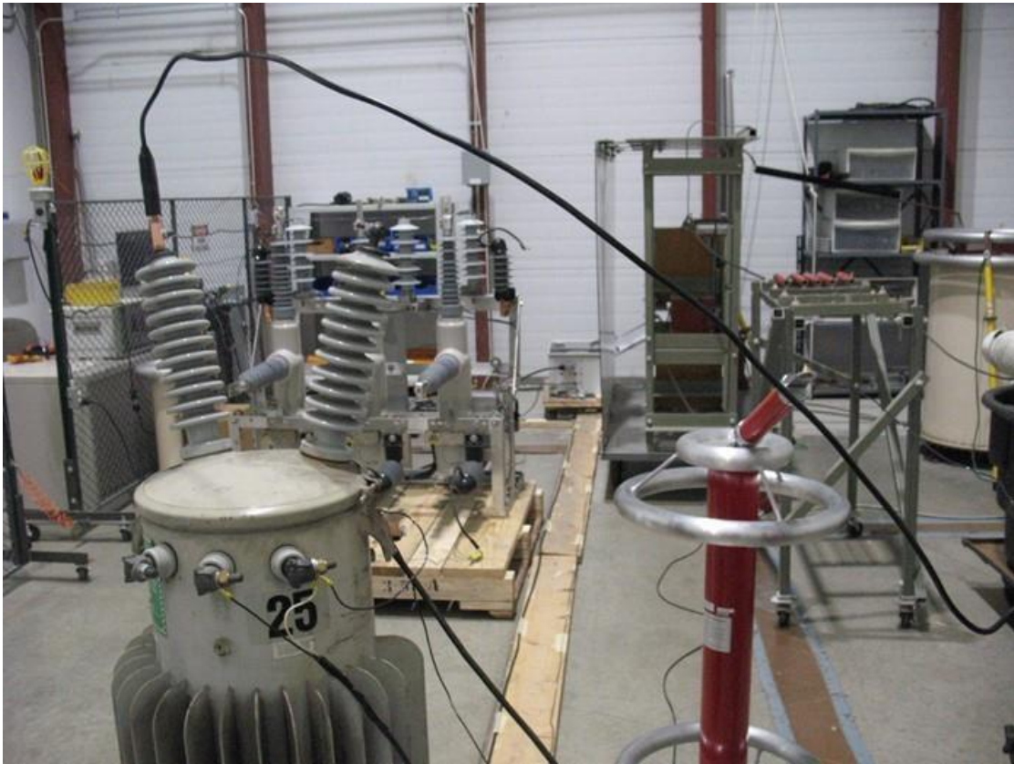
SSAO Transformer test setup
