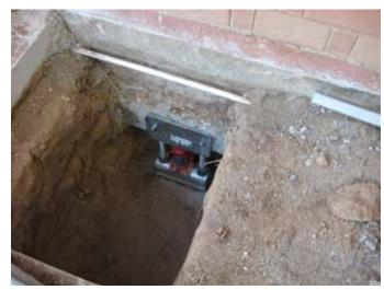
13. Apply a small amount of pressure to jack, just enough to take up the "slack" in the assembly. Once again check to see if the bracket is still mounted flush with the footing. Check the anchor mounting bolts again before proceeding.
