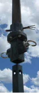
5. Assemble the lead section, extension, and Helical Pole Support together.
