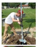
6. Insert the Drive End Assembly into the Helical Pole Support.
