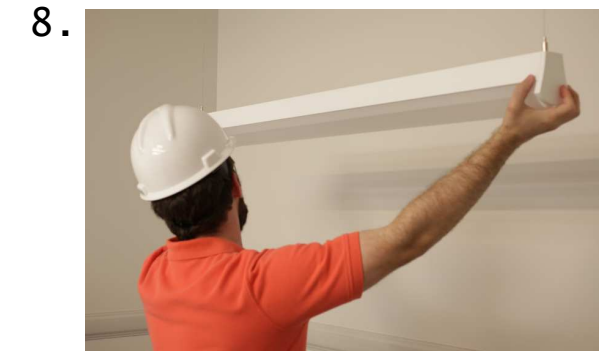
Pivot the lens into the housing around the end headers.
