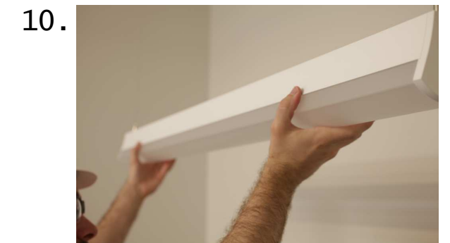
10. To ensure a secure fit and proper installation, feel along the seam between the lens and housing for any misalignment.
