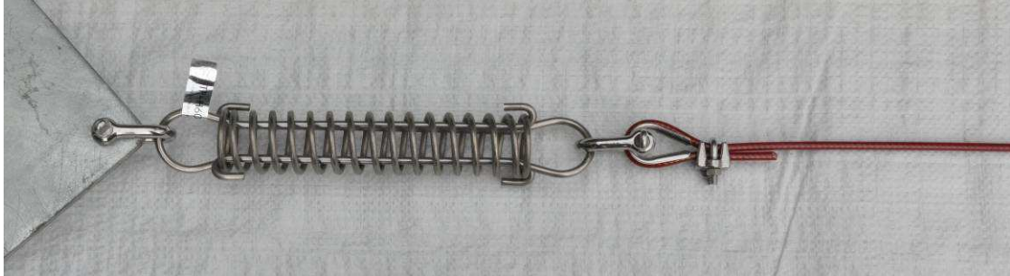
Photograph 7 Tension Spring Secured to Structure
