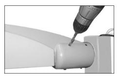
3. Remove slipfitter set screws, drill <sup>3</sup>/<sub>16</sub>" diameter recess in tenon for screw point and replace screws.
