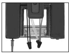
4. Caution: Structural integrity of mounting plate attachment to wall is by others. Securely mount wall plate cover assembly over wall plate and secure with screws. Connect wires observing polarity, i.e.: green-to-ground, white-to-common, and black-to-voltage.
