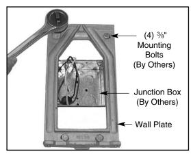
2. Securely mount wall plate over junction box (by others) on wall. Note: Hardware provided by others.
