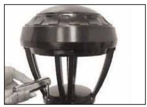
6. Install splice compartment cover with screws provided (2 places) using ½" hex wrench.
