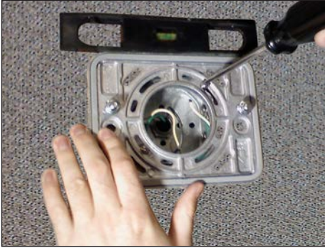
5. (WD14) Making sure plate is level and orientation arrow in pointing down, screw wall plate to 4" J-box with 8/32" screws provided, or to wall surface with 1/4" bolts (by others).
