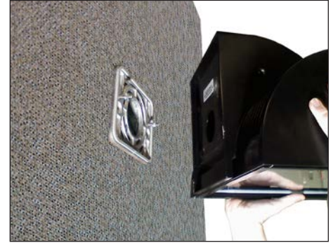
6. Hold fixture with both hands and guide keyhole slots on back of fixture housing onto mounting plate bolts, then slide fixture down.
