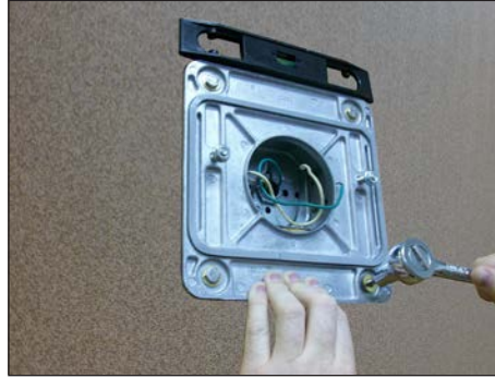
5. (WD18) Making sure plate is level and orientation arrow is pointing down, bolt plate to wall using 1/4" bolts (by others).
