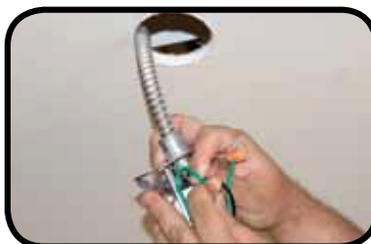
Pull the pre-existing wiring below the ceiling and connect to the J-tube assembly through the 1/2" knockout. A 3/8" flex conduit duplex connector may be used to easily daisy chain fixtures together. For end-of-run applications, a standard 1/2" connector can be used.
