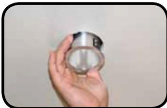
Squeeze retention springs, insert light engine assembly into the cut out, and push until springs pop out, and push until springs pop out above the ceiling, locking the fixture into place.
