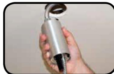
Simply slide the J-tube closed until it locks into place with the springs on opposite ends of the assembly to complete the third step.
