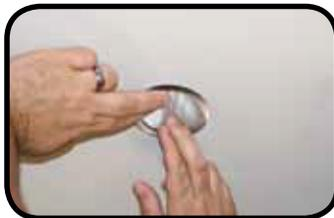
While the D2LED is designed with a life expectancy of over 50,000 hours, there may be times when you may need to access the fixture or J-tube assembly. For this reason, the D2LED has been designed to come out of the ceiling as easy as it went in.
