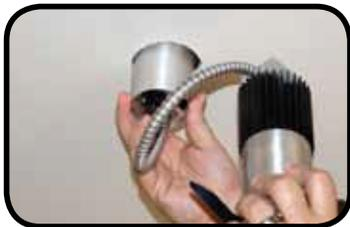
Feed J-tube assembly through ceiling cutout. The J-tube assembly has been designed to conveniently lay on top of the ceiling material. (NOTE: This fixture is designed for use in a non-insulated ceiling. See installed above ceiling view.)
